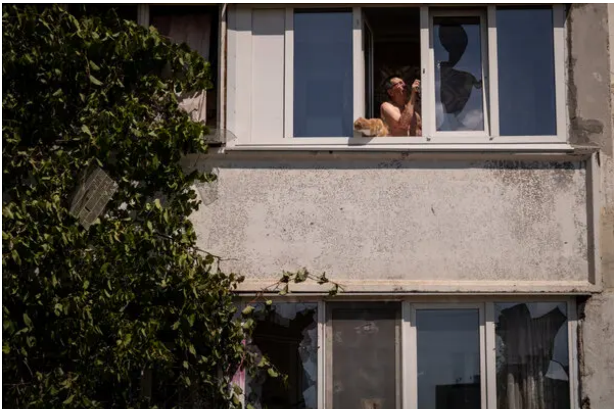
Removing shards of broken glass from the window of a residential building.
